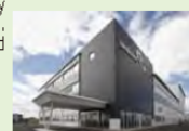
Technical Center and manufacturing facility for positive electrode material for lithium-ion batteries
